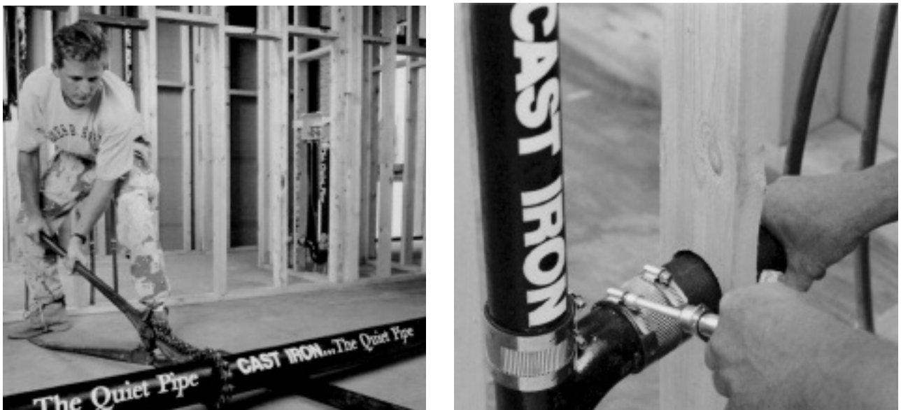
Figure 4—Assembling Hubless Cast Iron Soil Pipe Is Literally a Snap. Only Two Tools Are Required, a Pipe Cutter and Torque Wrench.
